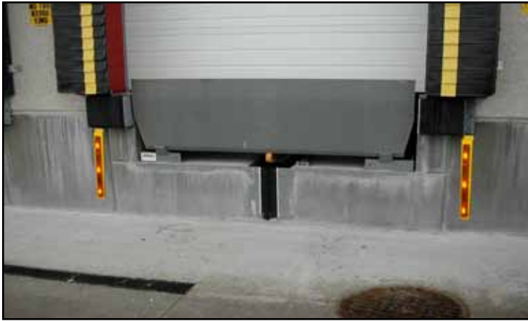
The LED guide lights allow truck drivers to easily see the bumper location and center themselves at the docks even in low light conditions
